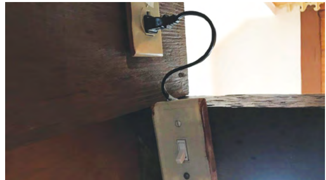
Picture 12: A flex cord supplying a light switch in an unapproved manner
